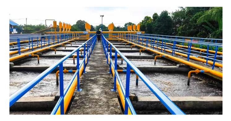
An effluent aeration system at the Halcyon Agri rubber processing plant in Jambi. Image by AWS Asia-Pacific
